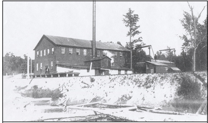
The toy factory in Casco, built by Edward Decker. Photo courtesy of KCHS photo collection.
